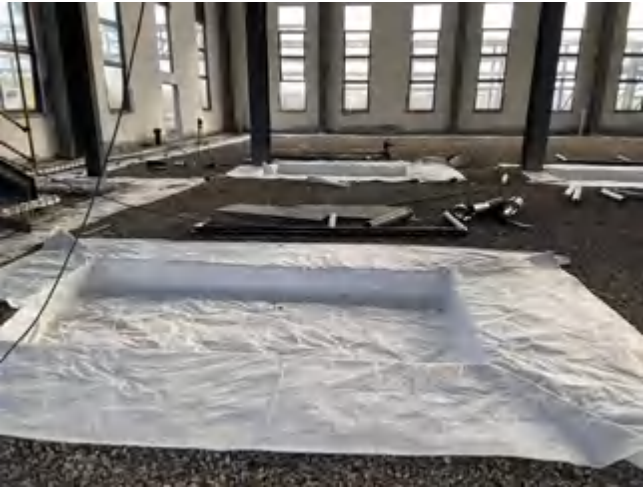
Feidong Gotion sets collecting ditches to avoid leaks
